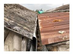
The guttering over the old kitchen in the south shed, has improved the water drainage off the roof, and much less rain seems to be getting into the building.
