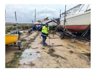
Some filling of potholes has been done with a team of "tampers" that spent time beating down the filling that was brought by dumper in the afternoon.
